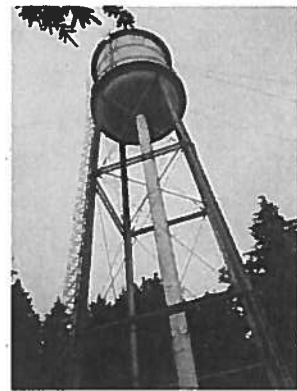
Beacon Hill reservoir
