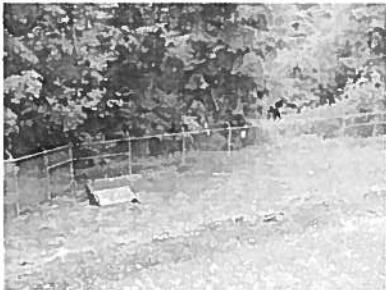
Altitude valve vault at Ostrander
