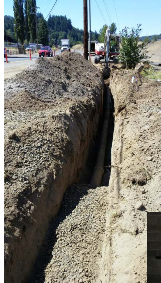
West Side Hwy Emergency Water Main Replacement
