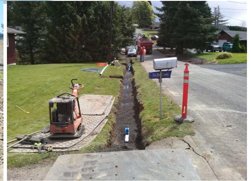
Crestline Place Water Main
