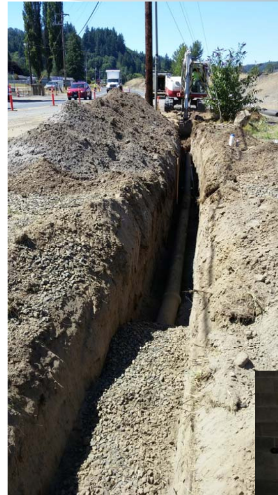
West Side Hwy Emergency Water Main Replacement
