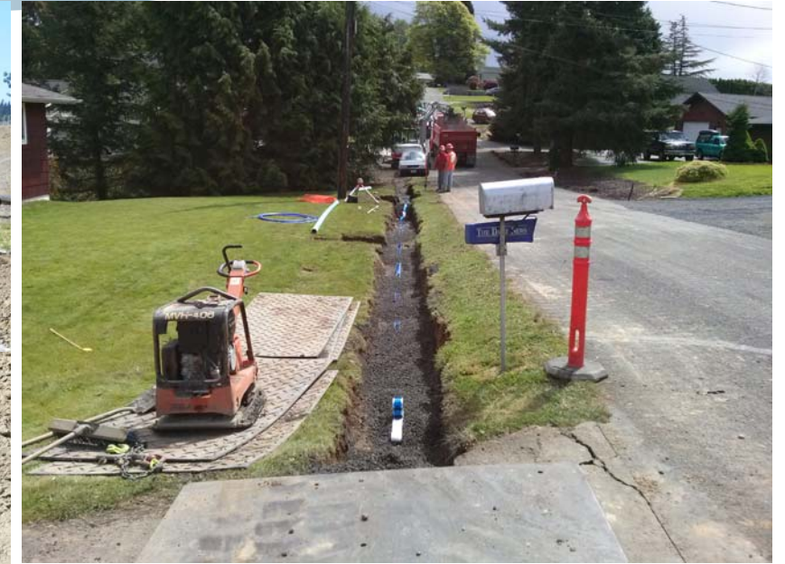
Crestline Place Water Main
